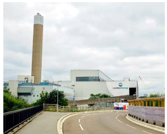
Figure 1: Waste incineration cogeneration plant in London, UK.
